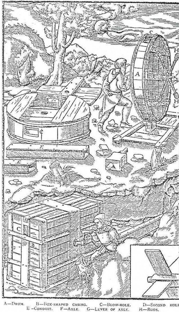
Fig. 4.18. A selection of mine ventilation fans. (4)
